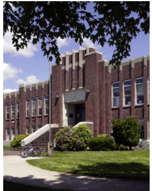
The Estacada Junior High School is a good example of a successful outcome, despite the inevitable challenges of a remodel.
