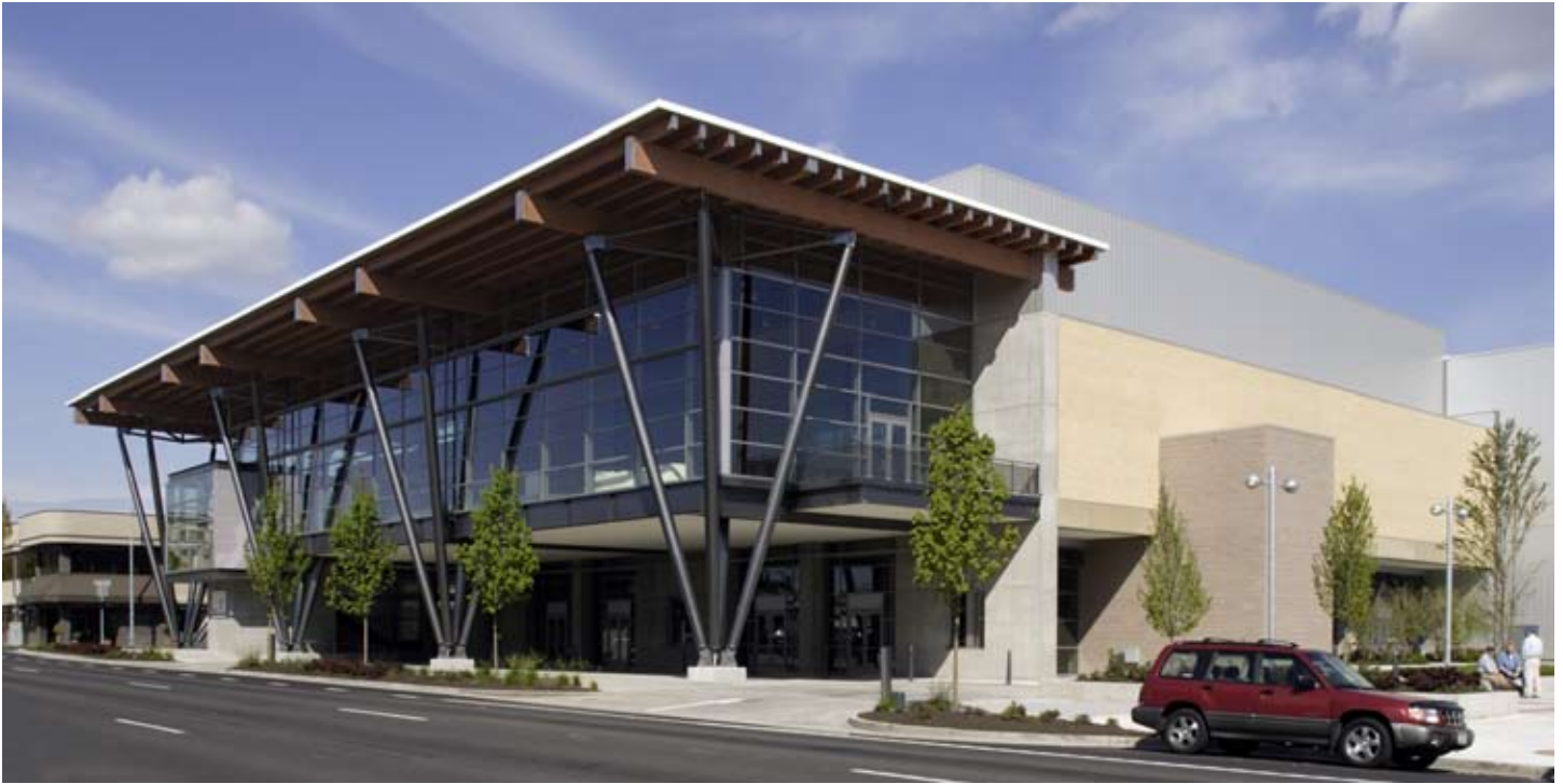
(Above) To address the effects of west-facing floor-to-ceiling glass, external awnings automatically open up and close, in response to the afternoon sun. This keeps the building cooler in summer and cuts air-conditioning use.
