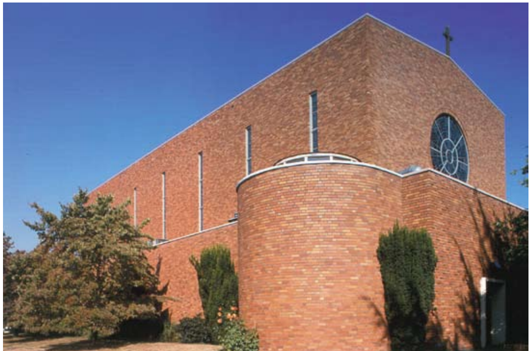
An historical wall of glass was reopened, allowing for daylighting and dimming controls.
