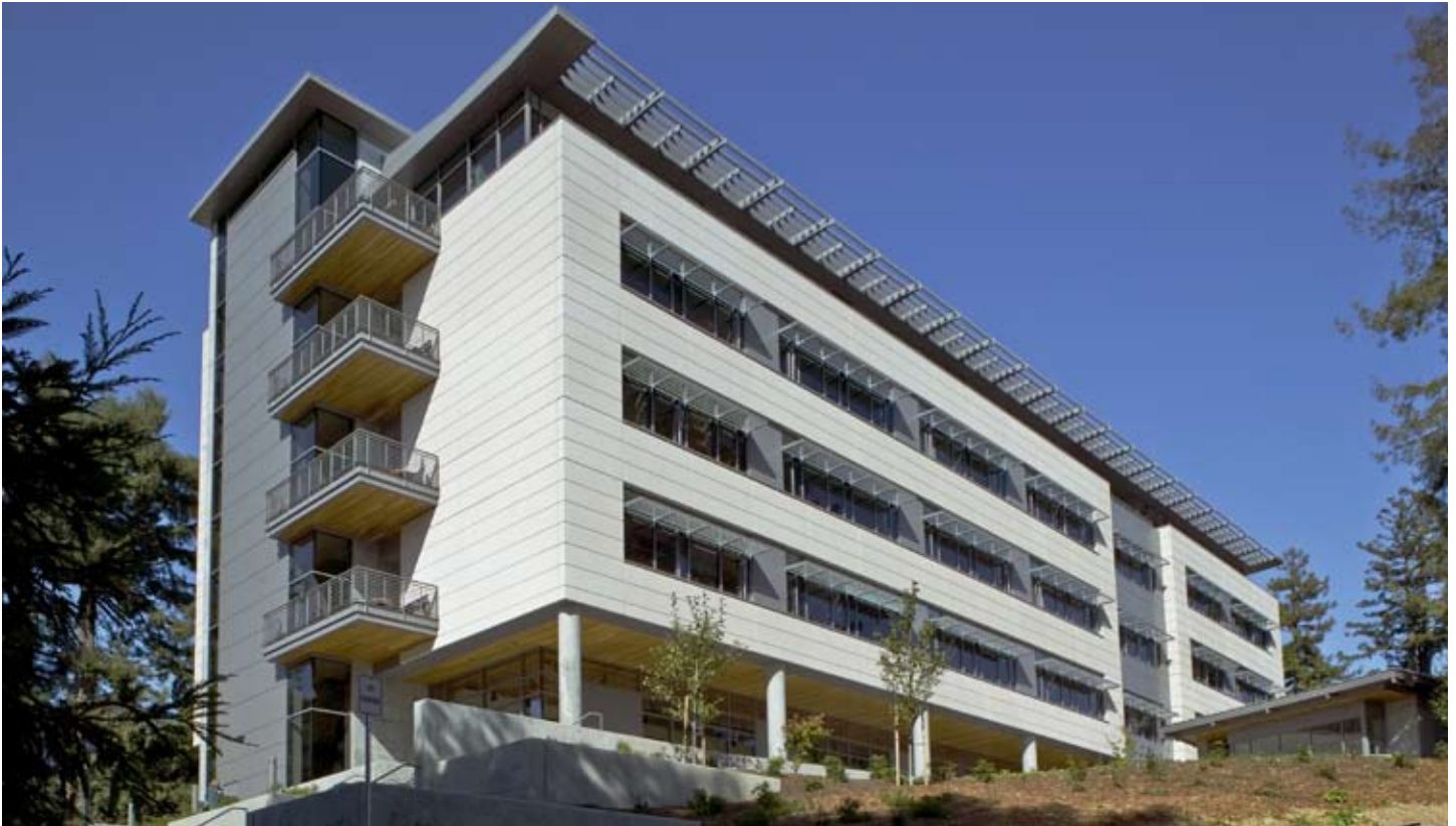
The Behavioral and Social Science Building expects energy savings exceeding 25 percent versus California's stringent new energy code. The facility will also capture 100 percent of on-site rainwater, using two 20,000-gallon storage tanks and a water treatment system.
