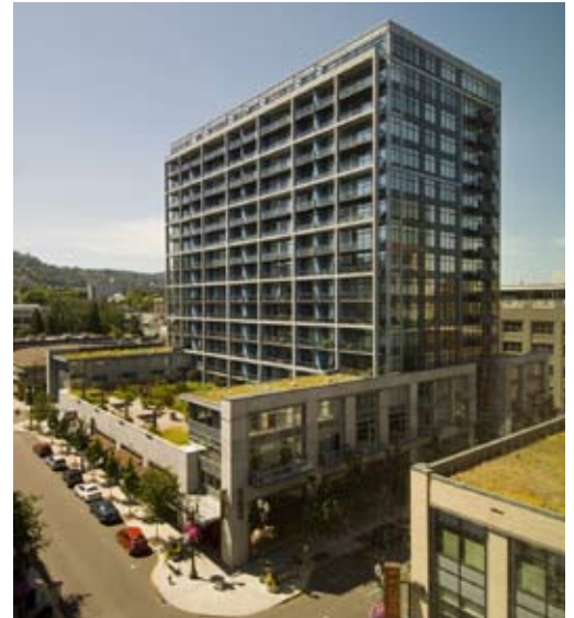
The building's operable windows allow for natural ventilation.
