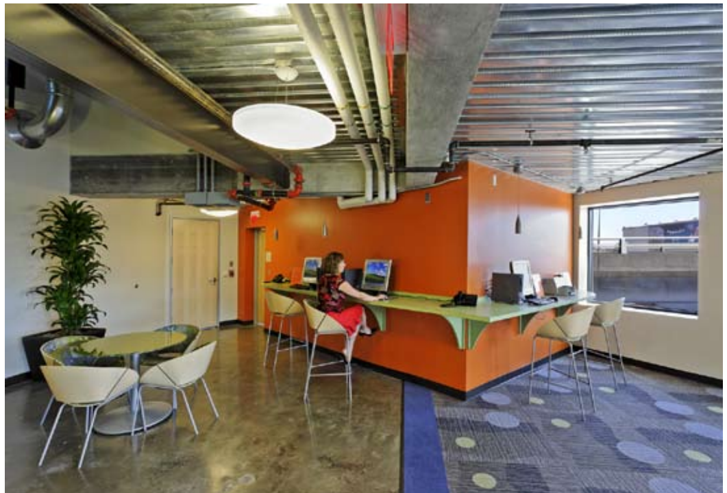
Interface Engineering used a track system to provide ambient lighting and highlight art work.
