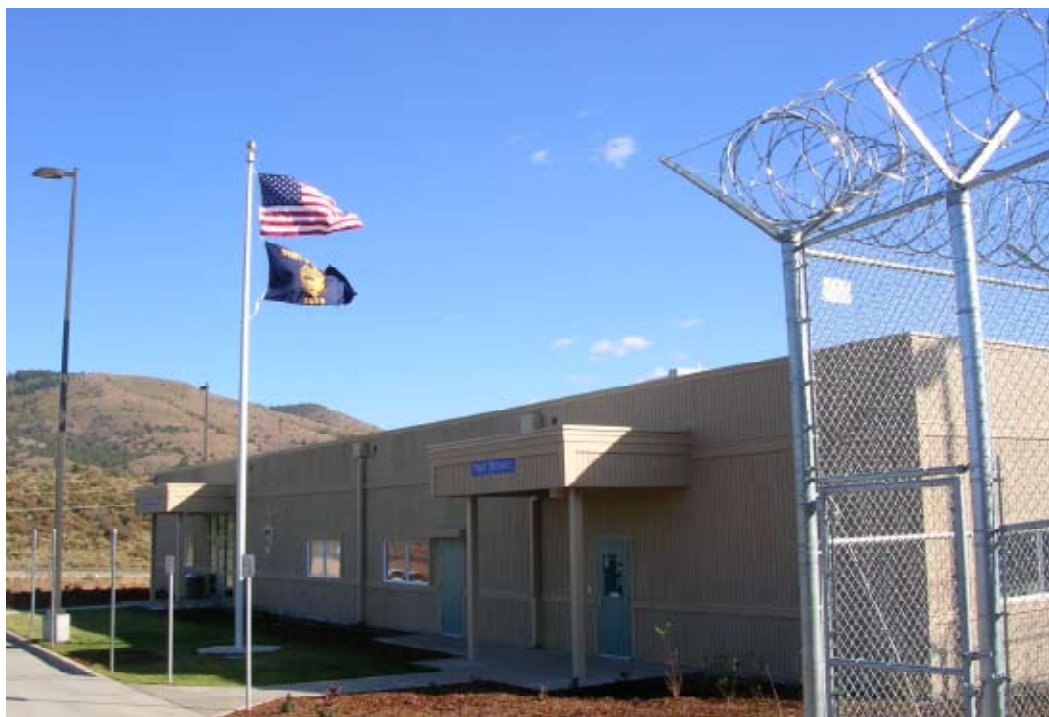
The correctional facility uses water from a 210°F geothermal heat source and, flowing through insulated pipes, arrives at the site at 200°F.
